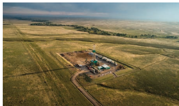
Commencement of operations at East Denver
